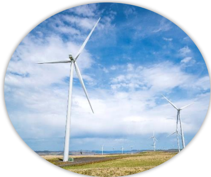
World-leading renewable energy development
